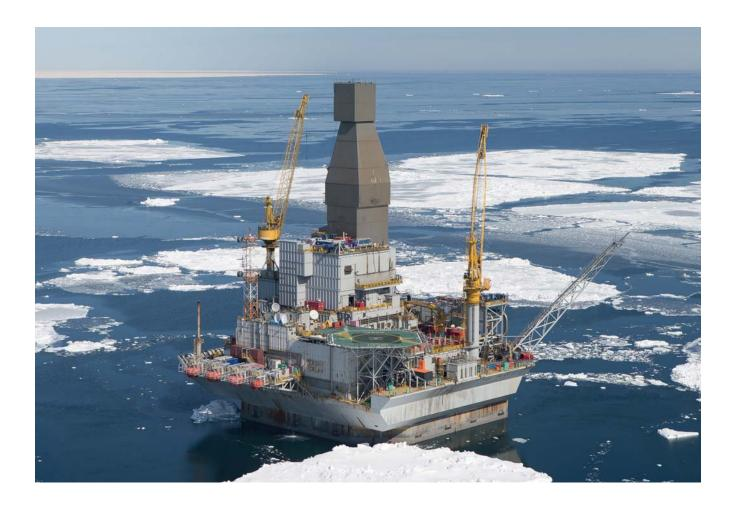
the southwestern and southeastern parts of the Chaivo field. Orlan's steel and concrete base is fit to resist ice and gigantic ice ridges rising up to a height of a six-floor house.
