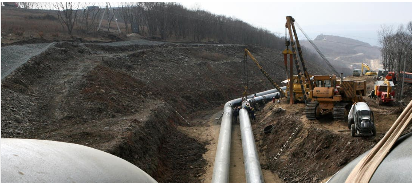
Construction of oil pipeline at Vankor
