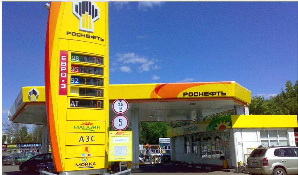
Filling complex #11 in Moscow
