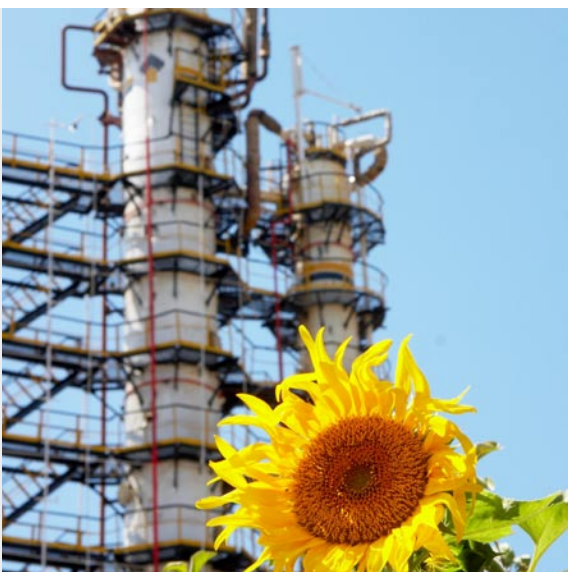
Gas fractionation unit #3 of Kuibyshevsk Refinery
