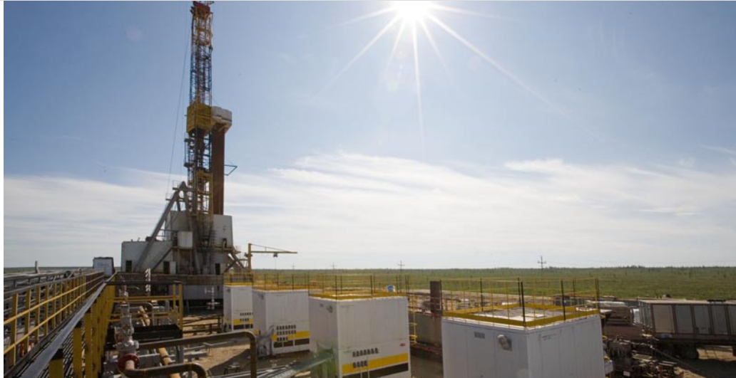
Wellpad #1 aof Vankor oilfield
